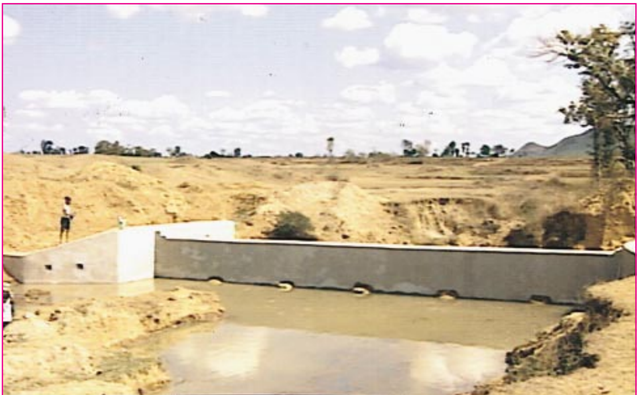
Protection Wall Developed under Watershed Programme
